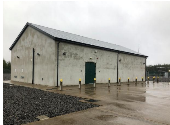
Plate 4-9 Substation Building 2 illustrating lack of bat access points.
