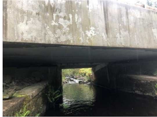
Plate 4-11 Underside view of bridge showing absence of features suitable for bat roosting.
